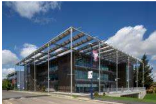
5G Innovation Centre building, University of Surrey
